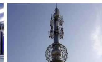
Telecom energy backup
